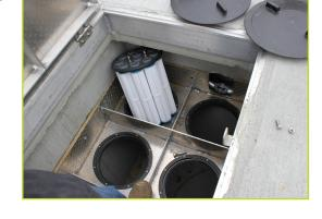
pretreatment and membrane filtration in a compact stand-alone solution. This combined treatment approach provide the needed water quality before sending clean, filtered water into the infiltration gallery, providing a long-term, smart approach to reduce maintenance costs and runoff volume.
